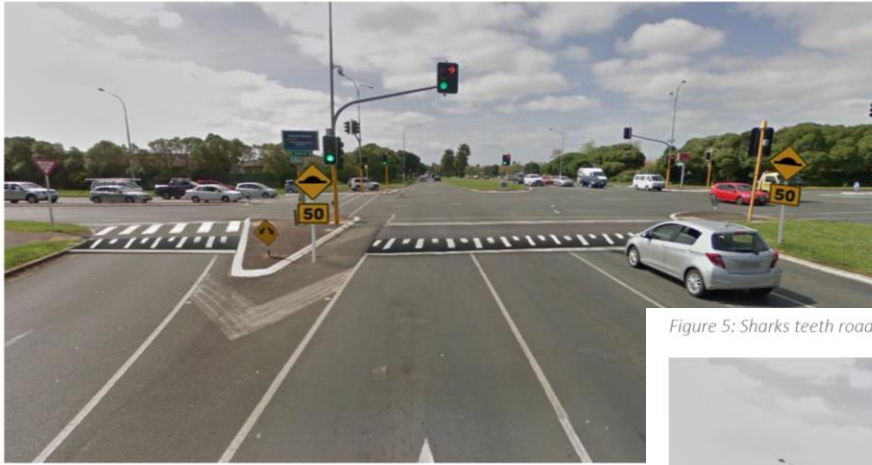
Figure 6: Piano keys road marking variation at intersection
