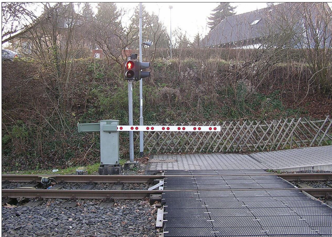
Figure 5-21: Example of pedestrian signals used with a barrier (Germany) (Wikimedia Commons)
