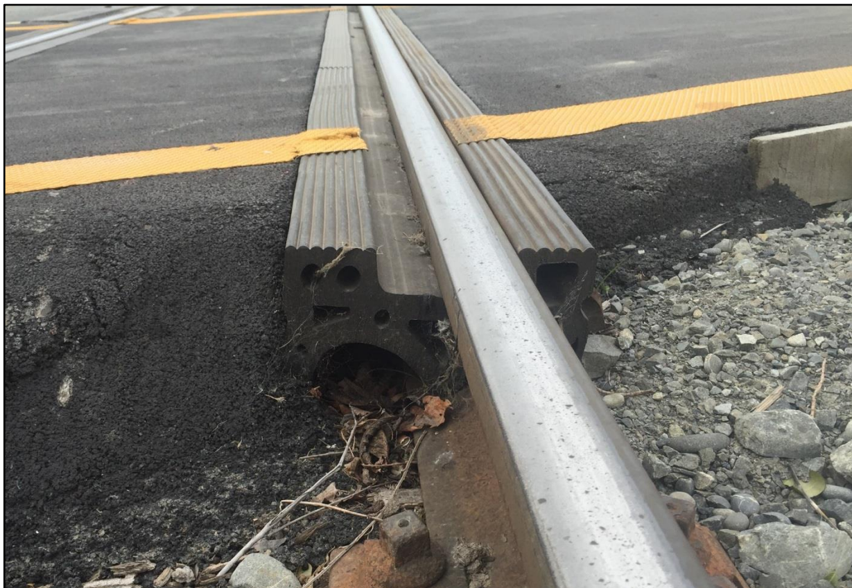
Figure 5-24: Epflex railseal used on asphalt railway level crossing (Kaiapoi)
