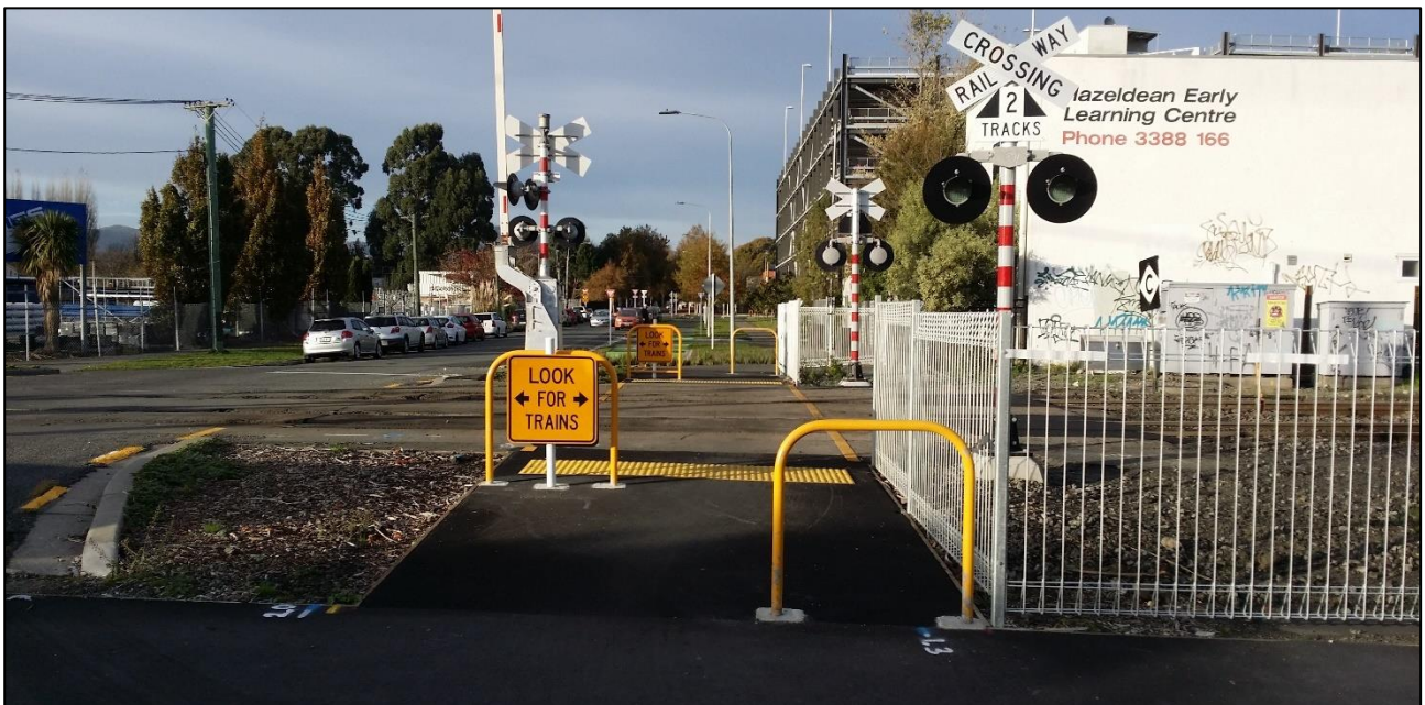
Figure 6-13: Example of alternating staples – Little River Link MCR at Grove Road, Christchurch
