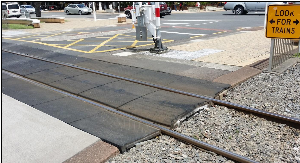
Figure 5-23: Rubber panel crossing treatment for road and path (CBD, Tauranga)
