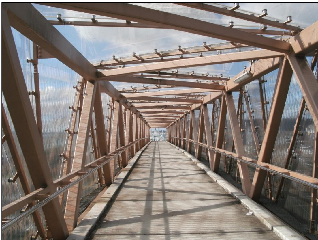
Figure 6-4: This overbridge features overhead and side protection from the elements (Auckland)
