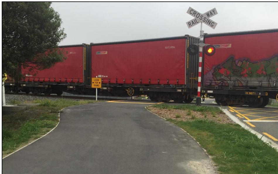
Figure 6-9: Flashing lights and bells on a path approach (Kaiapoi)
