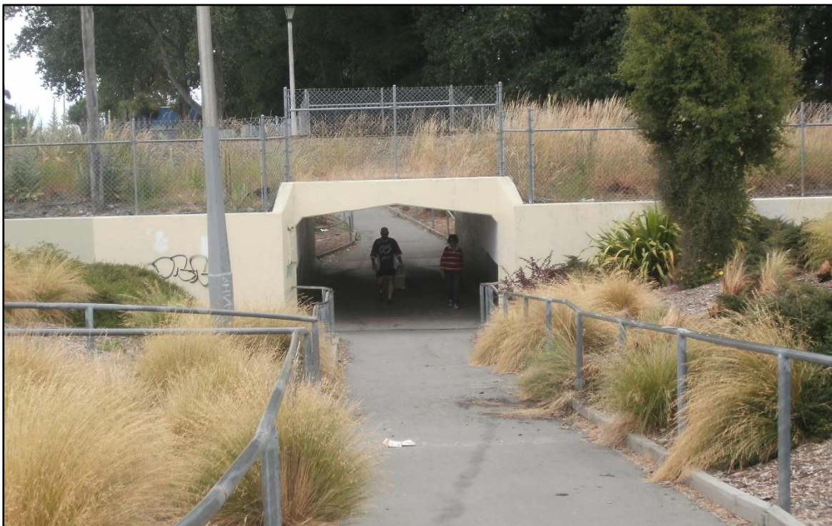
Figure 6-5: Railway underpass at Kyle Park with good sight lines, Christchurch
