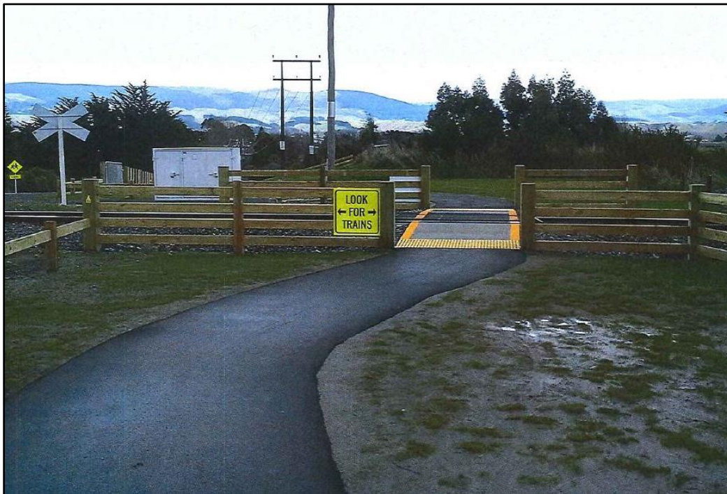
Figure 6-20: Unprotected crossing with minor chicanes and warning signs (Stoney Creek, Palmerston North)
