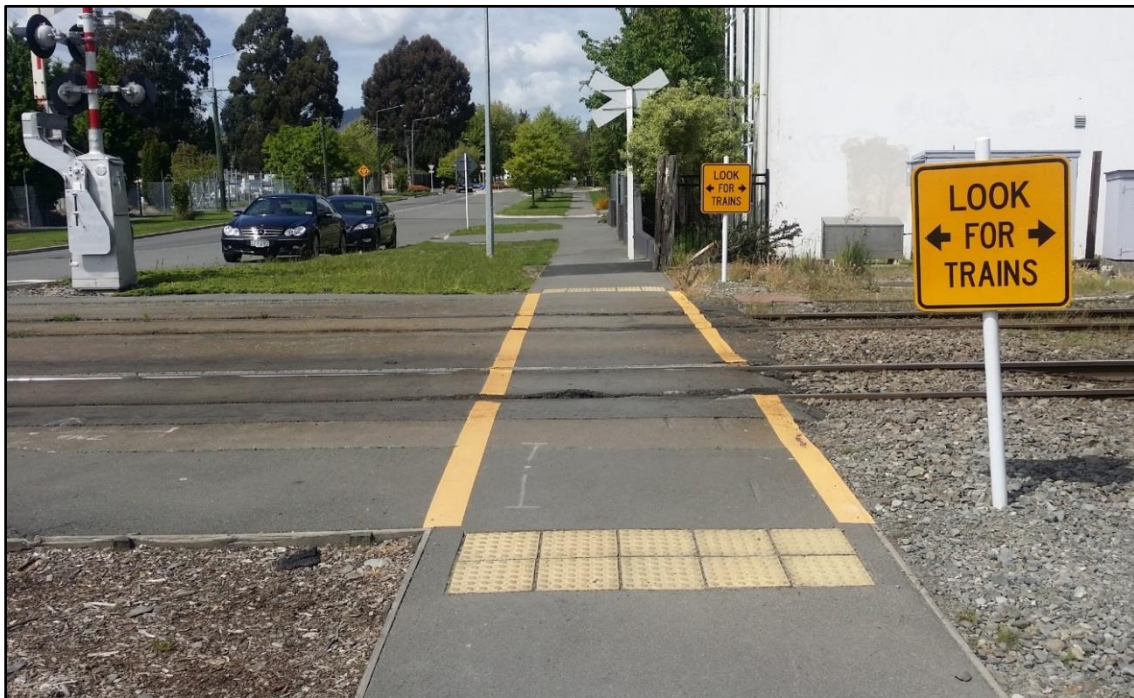
Figure 5-10: TGSi at level crossing - note no limit line applied (Grove Road, Christchurch)
