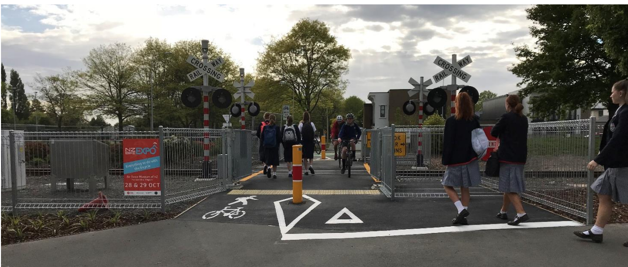
Figure 6-7: Double gate arrangement at Matai St level crossing, Christchurch
