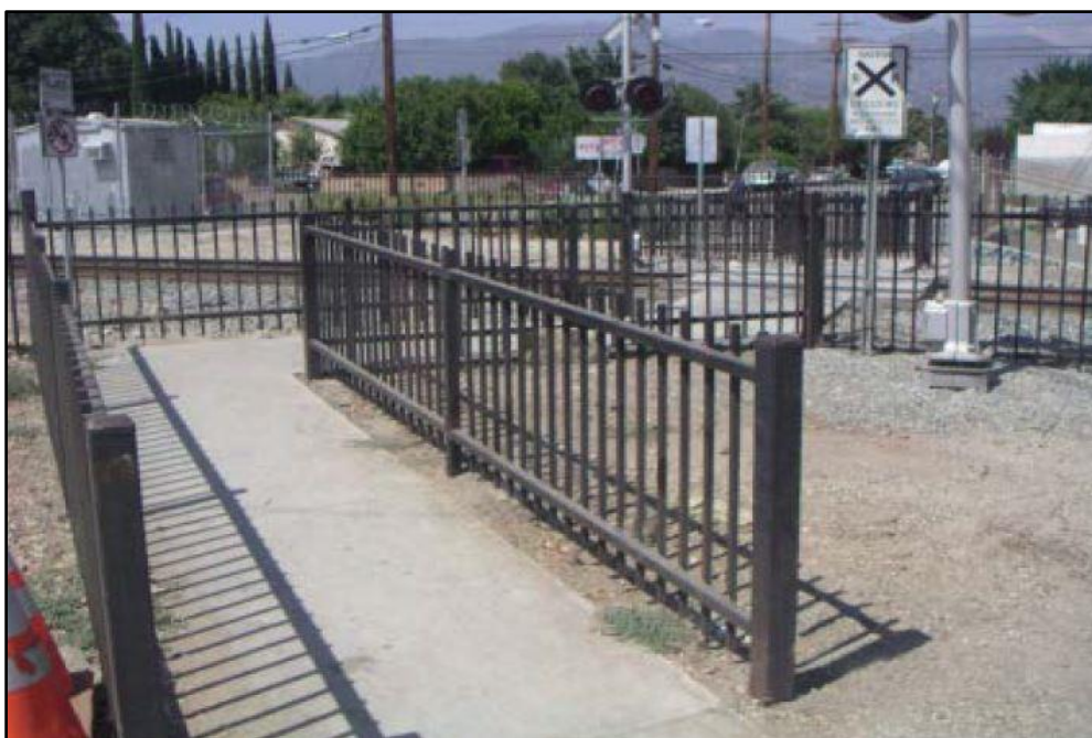
Figure 6-10: Example of a Z-crossing approach, albeit too narrow for easy cycle use (FRA 2016)
