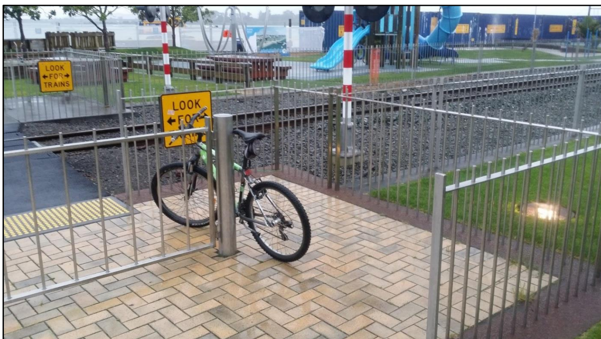
Figure 6-17: Consider the manoeuvre room available for a bicycle to get through a maze
