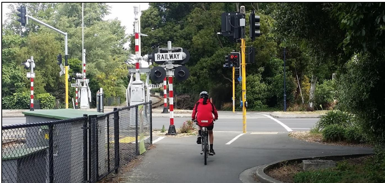
Figure 5-13: Fendalton Road signalised crossing adjacent to level crossing for road (Christchurch)
