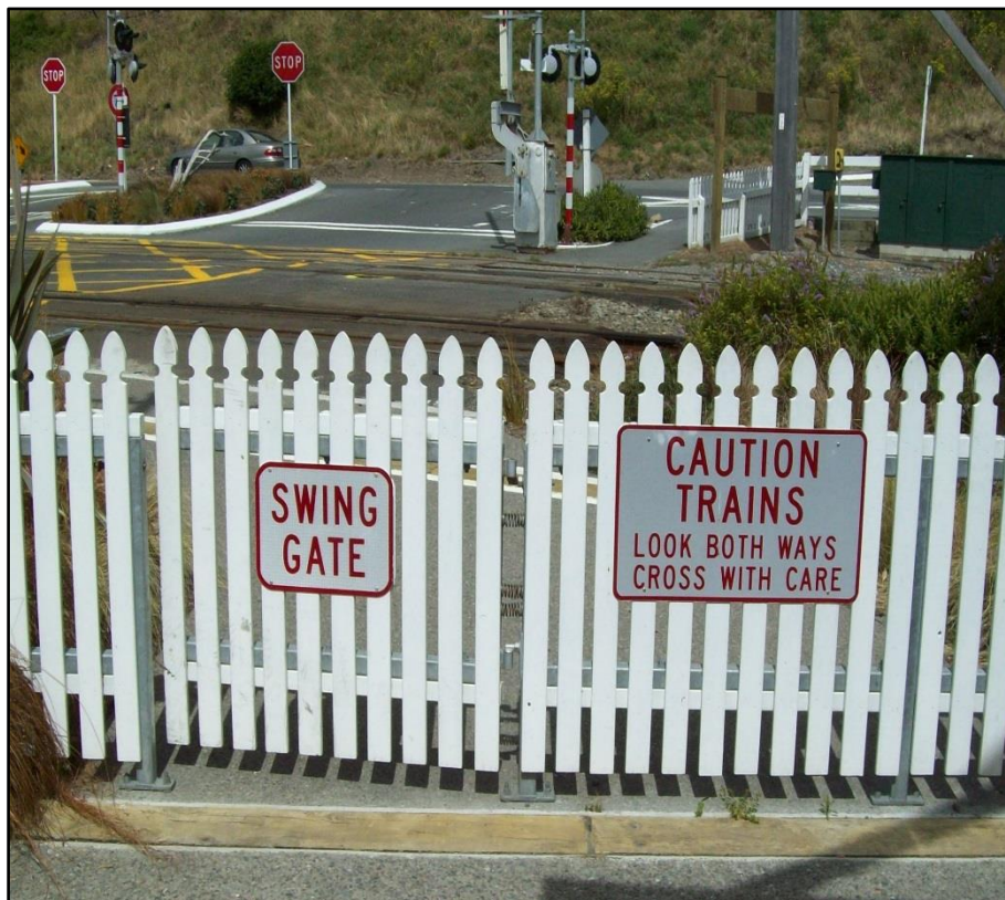
Figure 6-15: Manual swing gate at Beach Road (Paekakariki)
