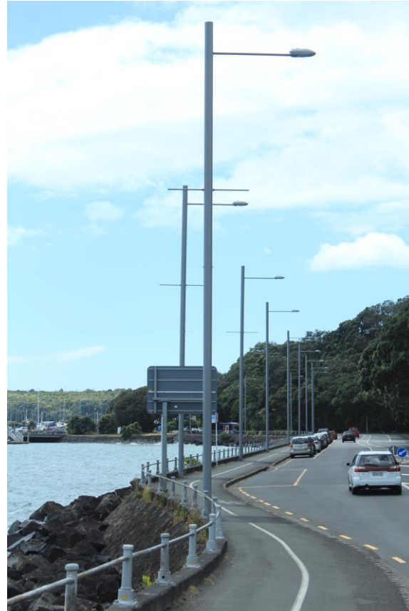
Decorative Streetlight Columns
