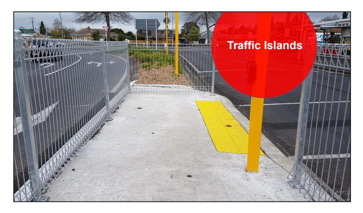
During the geometric design process the signals designer should be contributing to the design of traffic islands to ensure that they are in the right locations and the right size and shape for signals equipment to be installed on or for pedestrian facilities to be provided.
