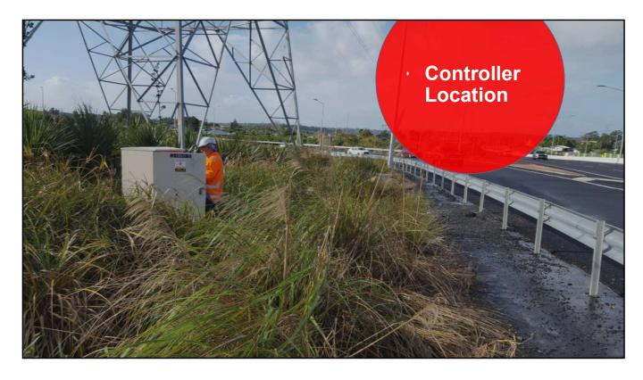
A suitable location should be included for the signals controller cabinet. It will have ducting running to it from the intersection which will include power supply to the poles, signal cabling and loop feeder cable from the detectors. It may also have communications cables. The location needs to consider all these underground connections in terms of utilities conflicts and power supply and the requirement for safe maintenance access.
