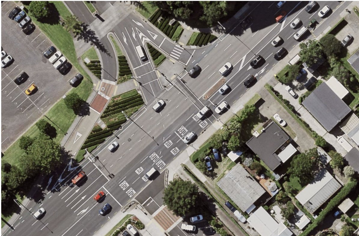
Figure 8-15: Historic signalised intersection layout – cycle lanes and continuity lines marked through intersection, contributing to red light running and crashes with side road traffic
