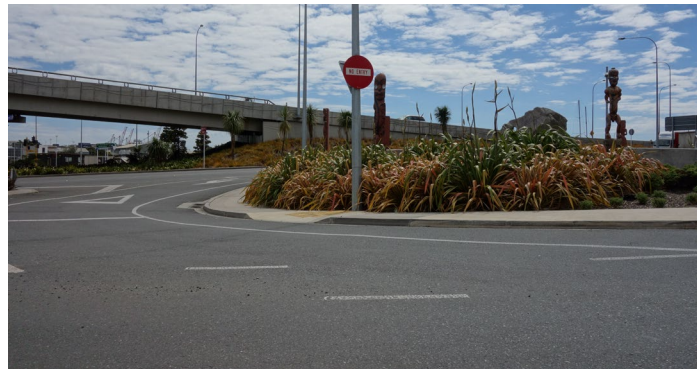
Figure 4-5: Pedestrian slip lane crossing point with poor visibility around the corner to approaching slip lane traffic
