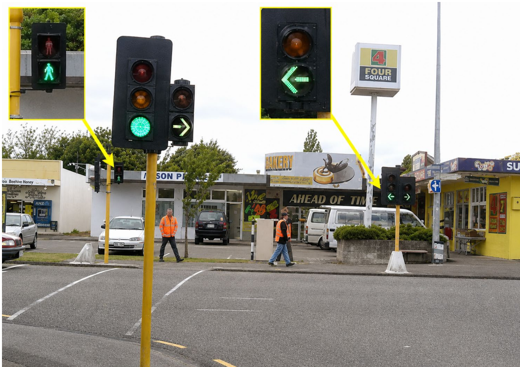
Figure 6-4: Dangerous ambiguity: walk and green left-turn arrow displayed simultaneously (original photo enhanced to improve resolution)
