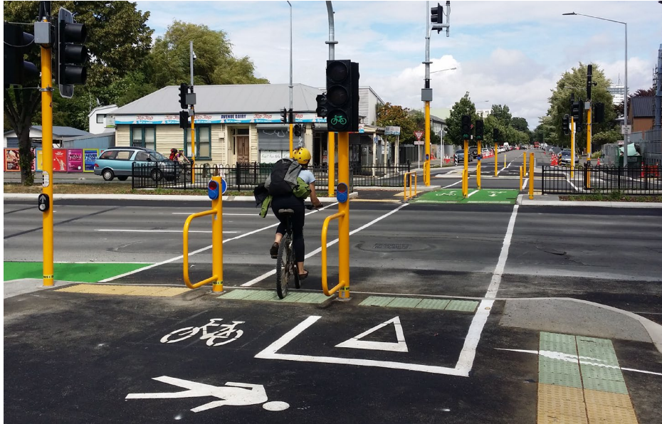
Figure 8-18: Midblock cycle crossing with call-accept lights (push buttons disabled)
