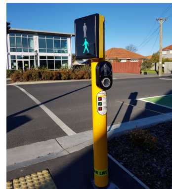
Figure 7-2: near-side pedestrian signals at midblock crossing
