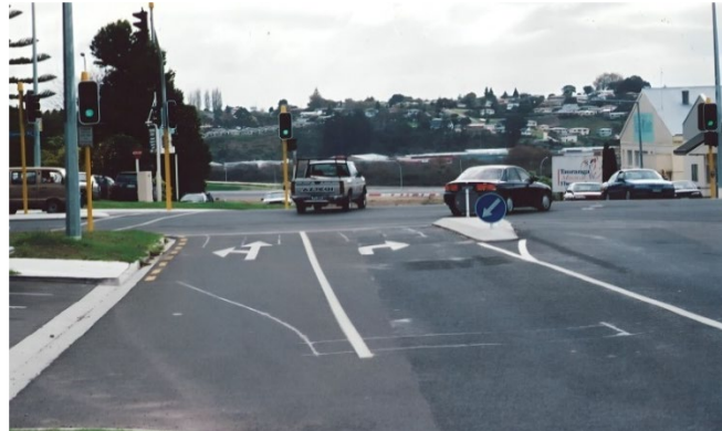
Figure 4-1: Offset right-turn bays with visibility issues (further restricted by vertical geometry)
