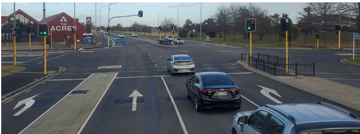
Figure 5-4: Fully protected right turn with the required three right-turn arrow displays
