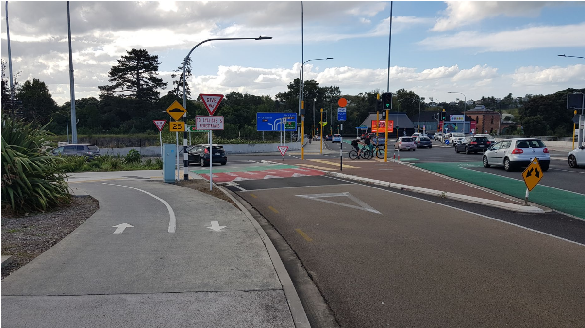
Figure 4-6: Slip lane with dual zebra / cycle crossing on raised platform for speed control
