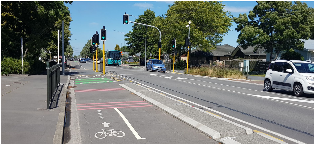
Figure 8-17: Cycle approach loops, marked with diamonds, approaching midblock crossing
