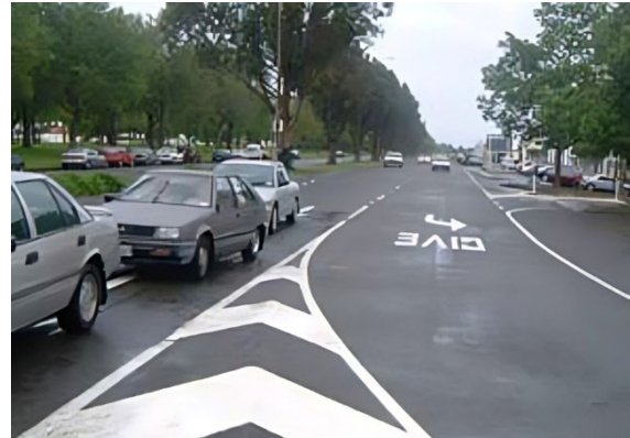
Figure 4-3: Historic example: captive left-turn lane with insufficient warning to motorists
