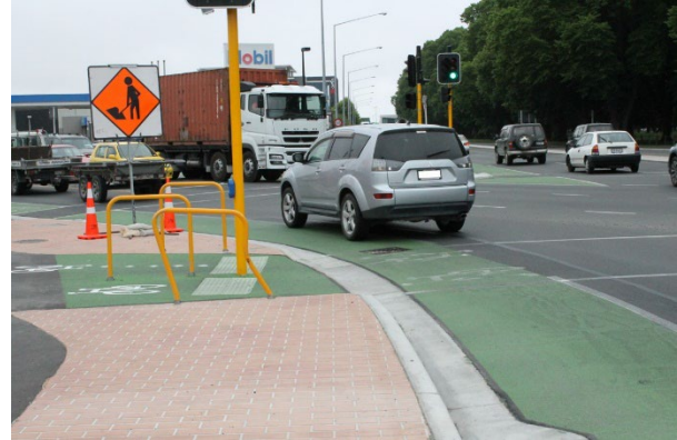
Figure 8-14: Car encroaching on cycle lane around bend through intersection
