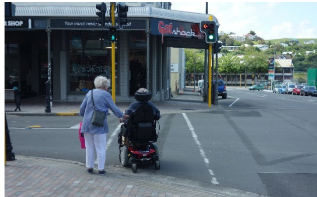
Figure 7-4: Poor provision – no pedestrian push button adjacent to crosswalk / cutdown
