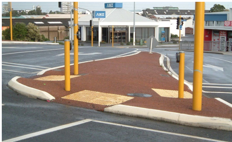
Figure 7-5: Use of stub pole for appropriate placement of pedestrian call box adjacent to the kerb crossing 2
